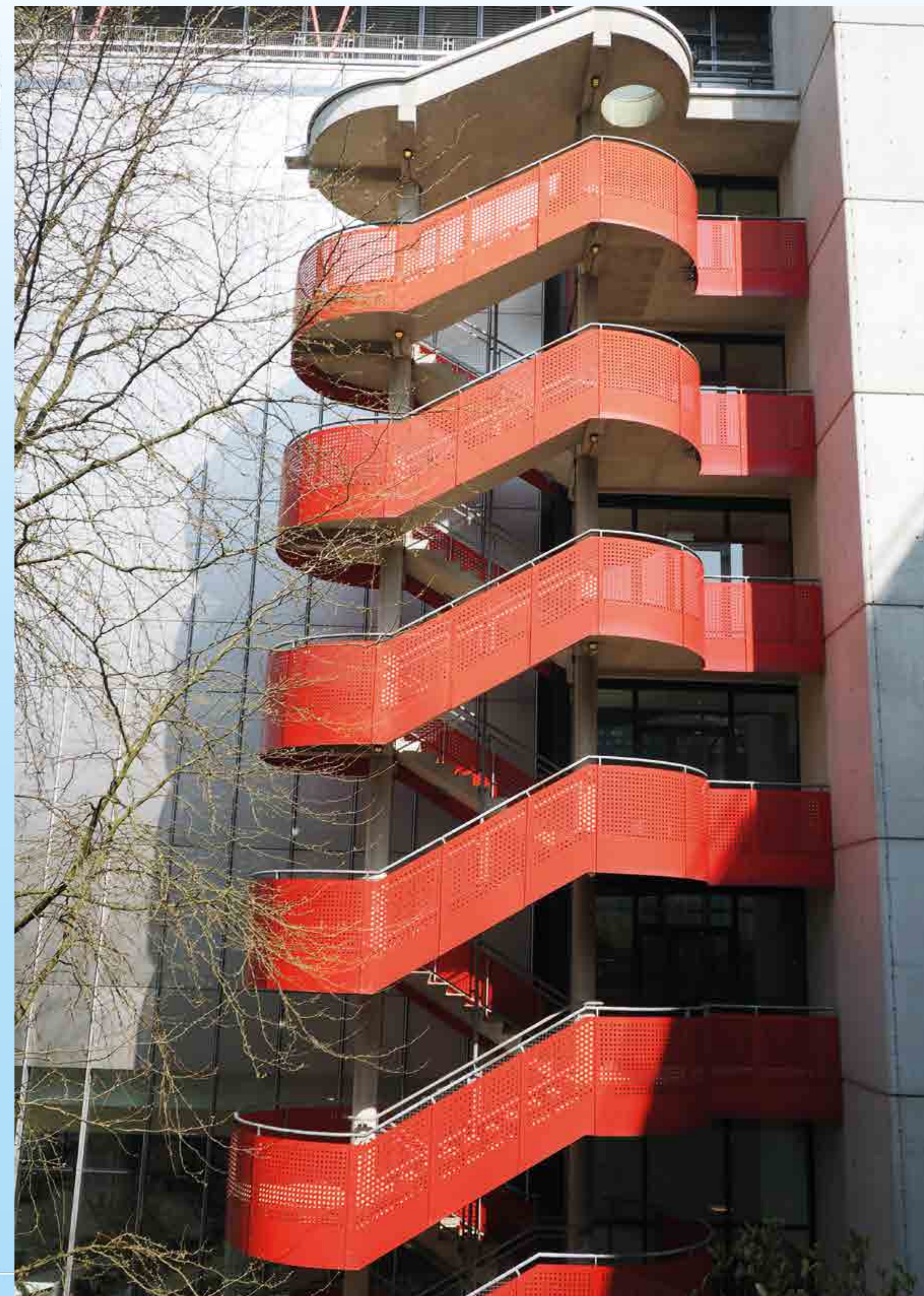
Staircase - where structure meets movement
