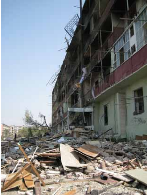
Bombed building in Gori, Georgia 29 September 2008. © Amnesty International
