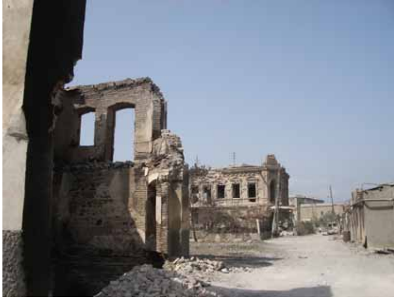
Ruined buildings on Thaelman Street in Tshkinvali, South Ossetia, 29 September 2008. © Amnesty International
